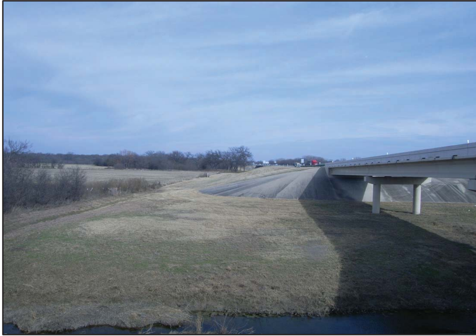
Photograph 5: View looking northeast towards the Catherine Branch from the IH 35W west ROW near STA. 240+00. Date of photograph: 12/8/19.
