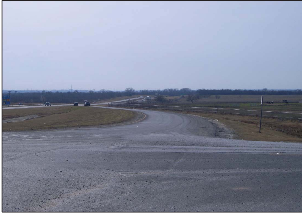
Photograph 9: View looking south towards IH 35 W west from the FM 1171/ Cross Timbers Road ROW near STA. 330+00. Date of photograph: 12/8/19.
