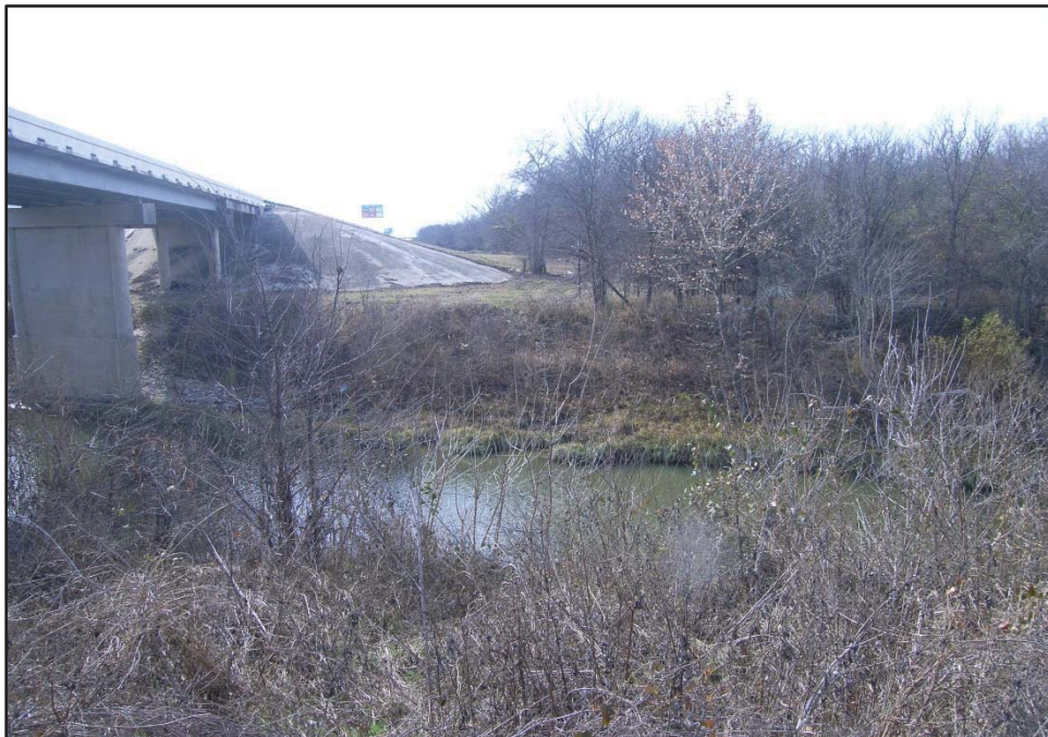
Photograph 6: View looking southwest across Denton Creek from the IH 35W west ROW near STA. 277+00. Date of photograph: 12/8/19.
