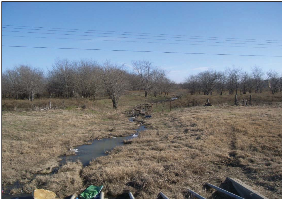
Photograph 8: View looking east southeast towards the Cleveland Branch from the IH 35W east ROW near STA. 300+00. Date of photograph: 12/7/19.
