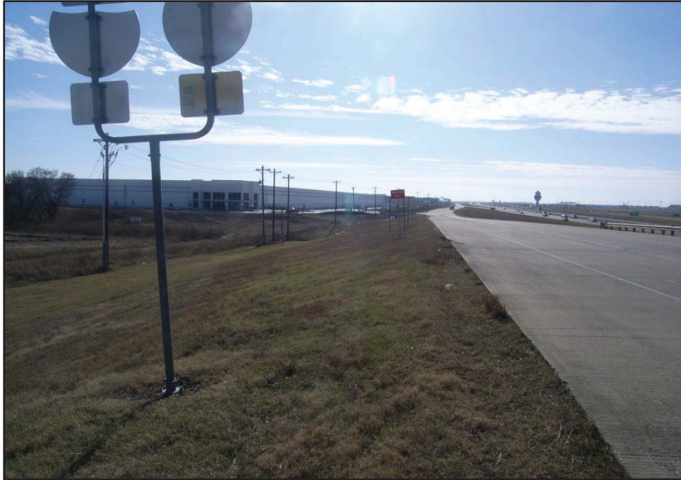
Photograph 1: View looking south along the IH 35W northbound frontage road near STA. 229+00 at the southern project terminus. Date of photograph: 12/7/19.
