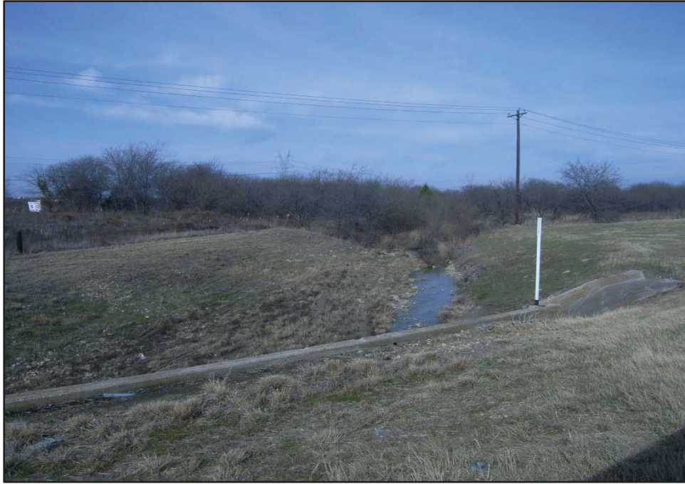
Photograph 11: View looking northwest towards Graham Branch from IH 35W west ROW near STA. 520+00. Date of photograph: 12/8/19.
