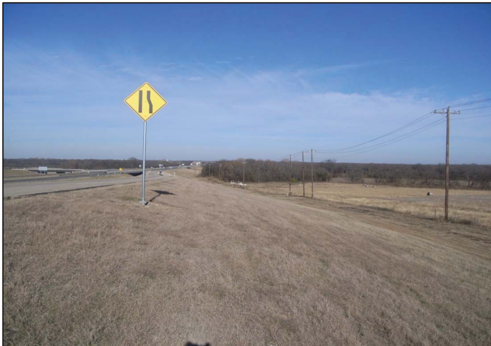
Photograph 2: View looking north along the IH 35W northbound entrance ramp near STA. 229+00 from near the southern project terminus. Date of photograph: 12/7/19.
