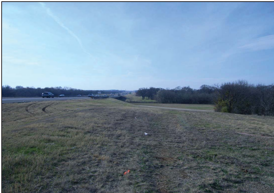
Photograph 18: View looking southwest towards Corbin Road from the IH 35W west ROW near STA. 825+00. Date of photograph: 12/7/19.
