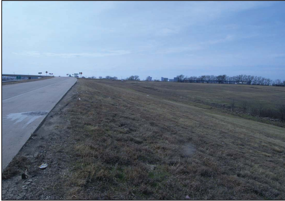
Photograph 3: View looking west southwest along the southbound IH 35W exit ramp to Dale Earnhardt Way. Date of photograph: 12/8/19.
